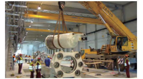
Transfer and installation of extrusion presses
